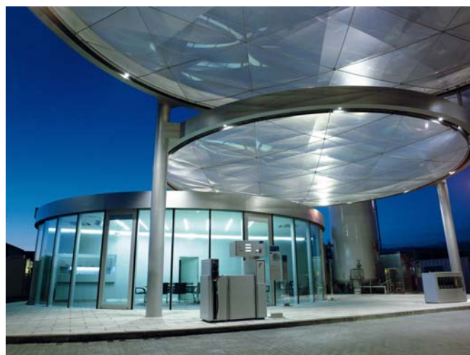
The Linde Hydrogen Center near Munich – photo courtesy of The Linde Group
